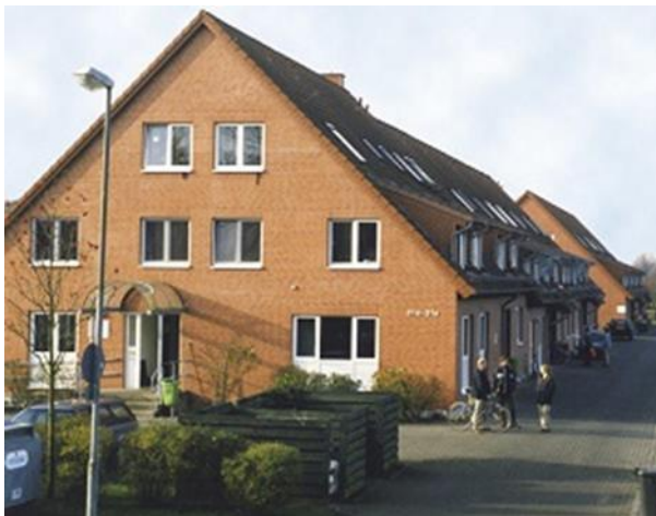
student dormitory "Estebrügger Strasse"
